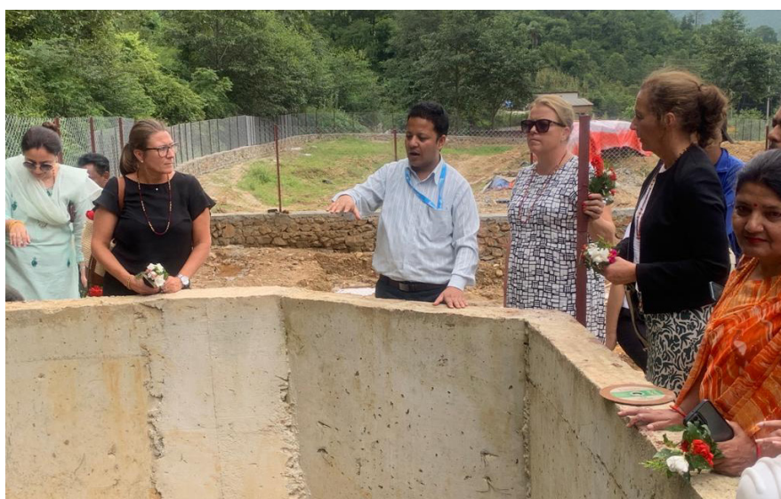
Swedish parliamentarians visit at the construction site in Lele.
